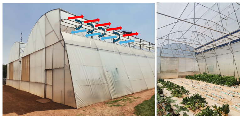
Figure 1: (left) CEI Agrihub Sawtooth greenhouse at University of Johannesburg. Note the vents which form part of the aerodynamic roof shape. The swirls represent vortices that bring cool air into the greenhouse and flush out hot air, which is represented by red arrows, to the outside. (right) Internal structure of the greenhouse with various crops within the greenhouse.
